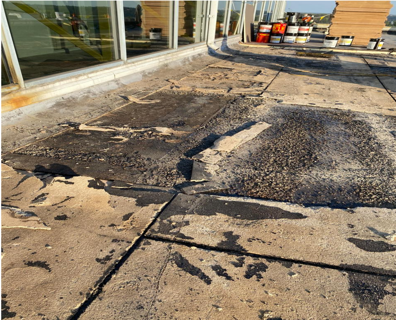
ASB Building Before
