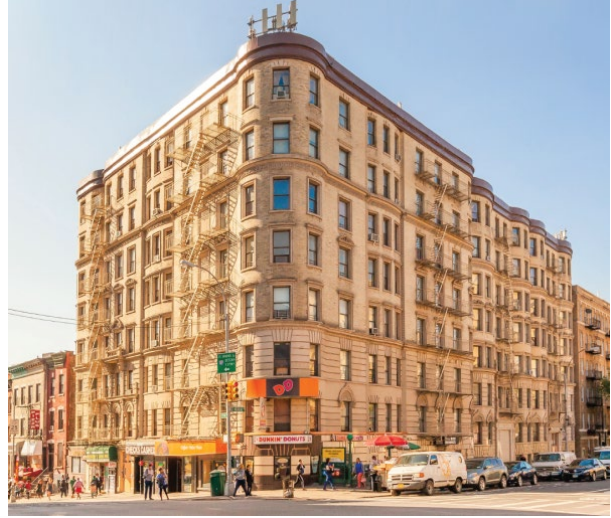
St. Nicholas Manor | Manhattan, NY | 112 units | Section 8
