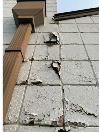
Paint and CMU spalled adjacent to through wall conductor head. Typ at most conductor head location, especially along South Facade
