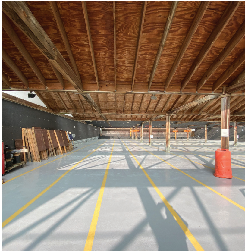
Underside of plywood roof deck
