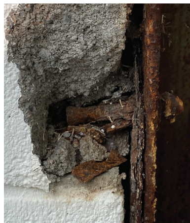
Overhead door track anchors are all heavily corroded and spalling caused adjoining CMU to crack and chip away
