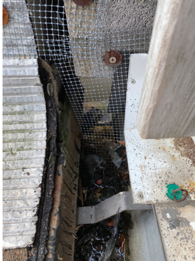
Gutter through-wall opening at expansion joint, which is allowing water infiltration into CMU wall, note joint is completely open on back side
