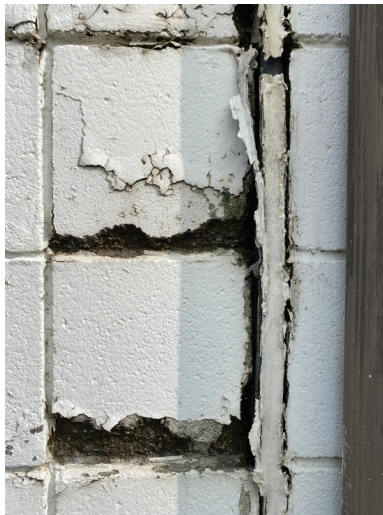
Enlarged image, lower section of expansion joint
