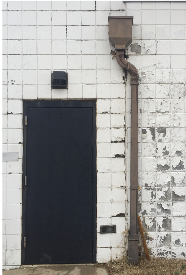
Severe deterioration at control joint
