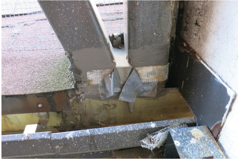
Gutter & through-wall scupper
