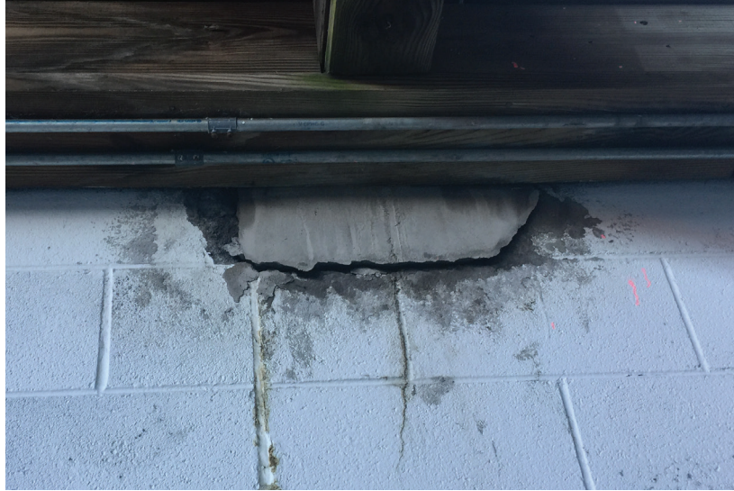
Failing CMU beam pocket repair
