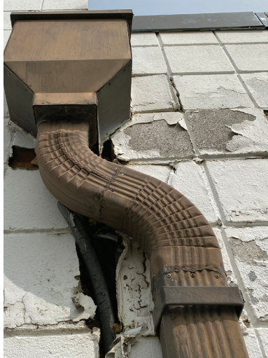
Enlarged image, exposed expansion joint and failing CMU at through-wall scupper
