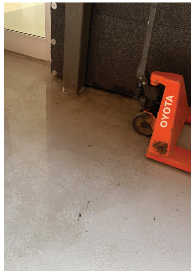
Ponding water on floor slab, due to leaking gutter and wind driven rain. Could be trip hazard through formation of ice in winter
