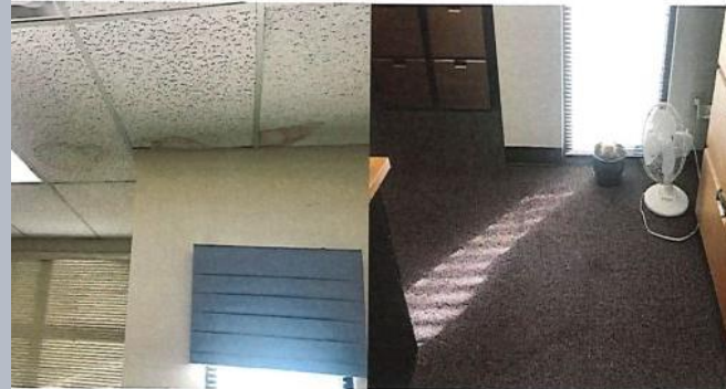
15 - Outside Office / Reported leaking under heavy rain
