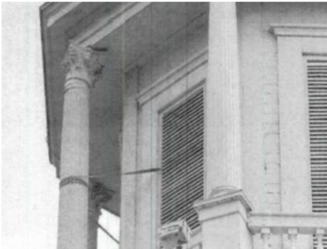
Damaged rear belfry column.
