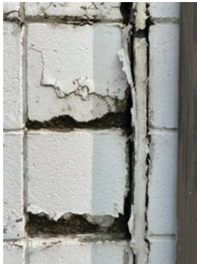
Enlarged image, lower section of expansion joint
