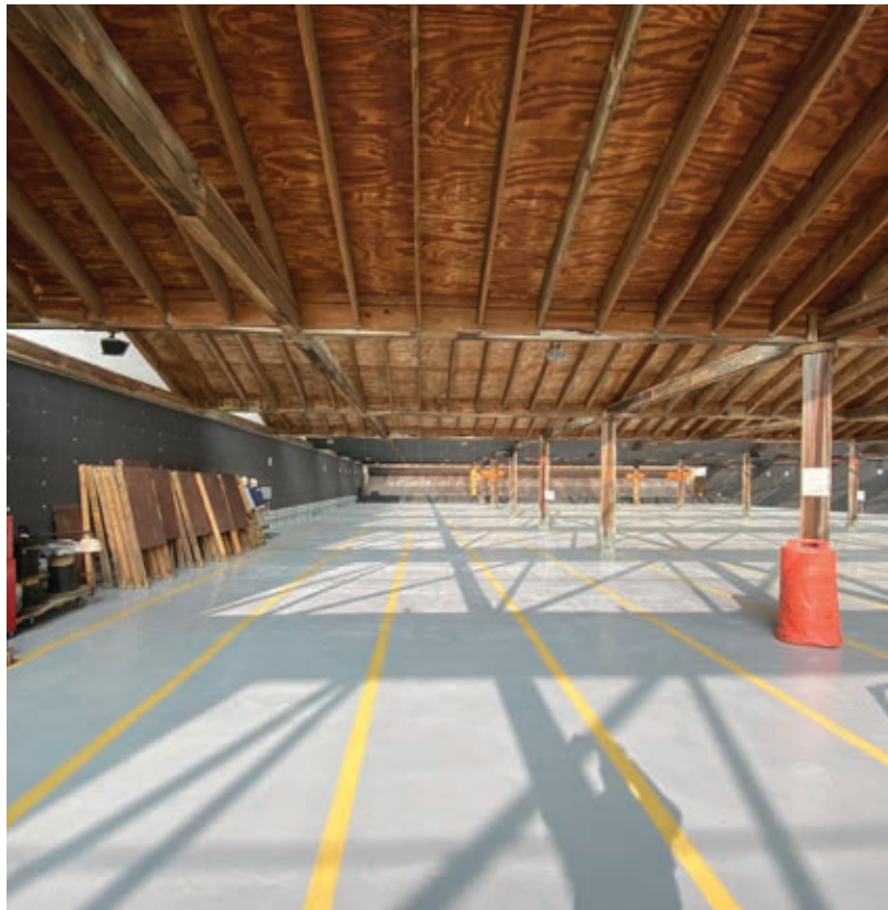
Underside of plywood roof deck
