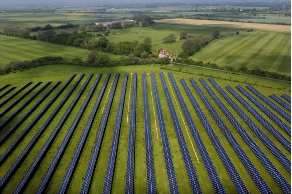
Romney Marsh Solar Farm in the U.K., which provides enough power for around 6,000 households. PHOTO: GARETH FULLER/ZUMA PRESS
