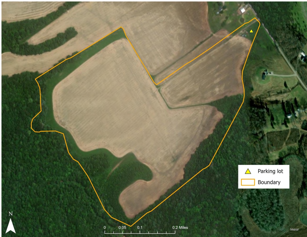
Figure 33: Possum Hollow 2024 IPBI/Maintenance Area
