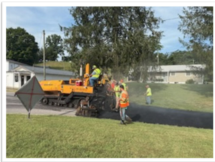
Photo 1. RMA Paving Project, Crocus Road, Russell County Photo by Jon Durbin
