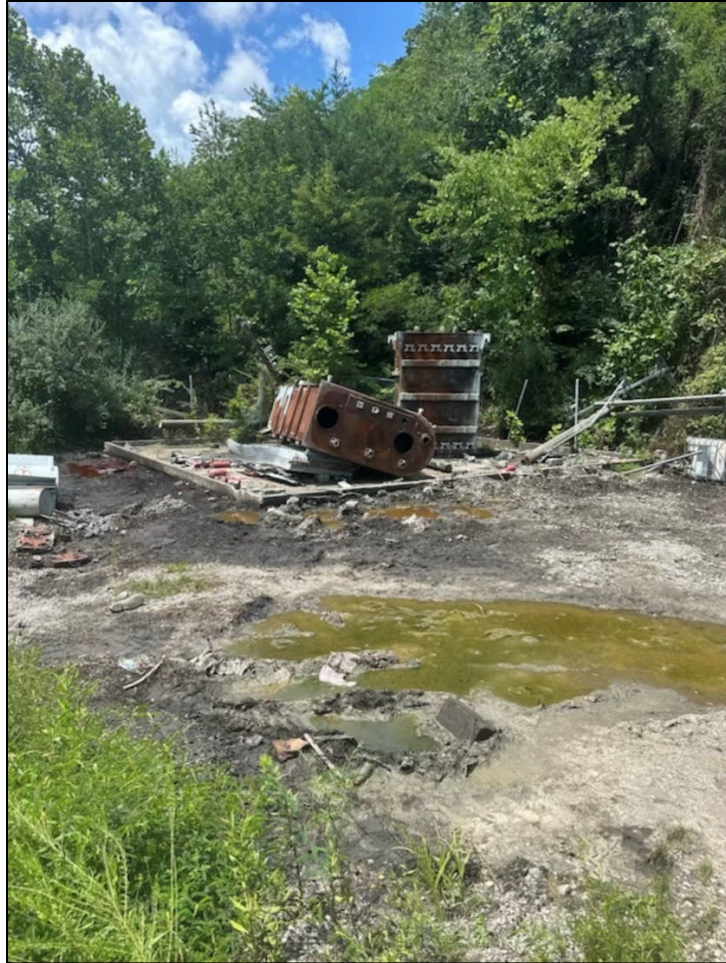
Photo: Non-PCB transformer oil spill at former Revelation Energy site.
