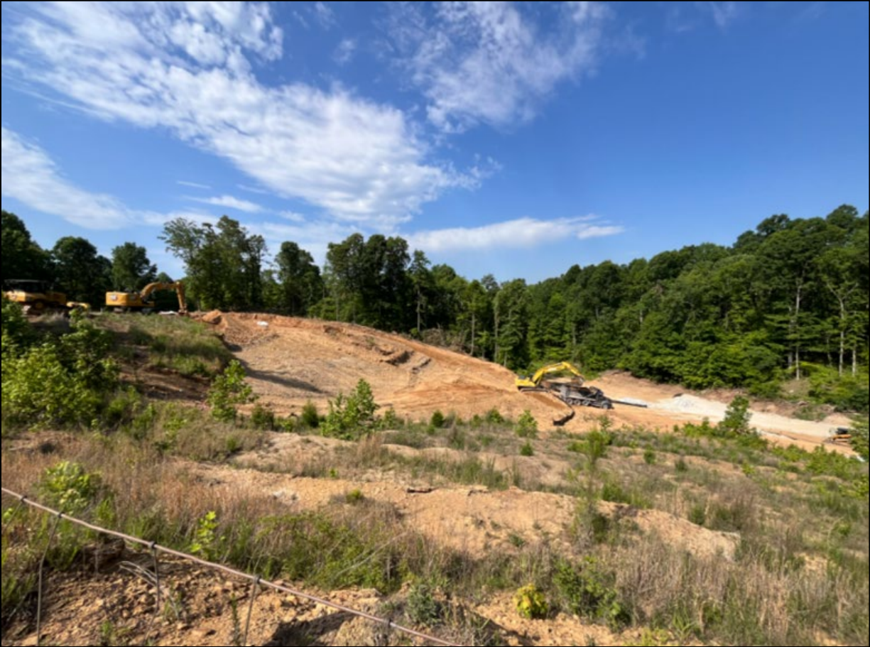
Photo: Excavation activities currently taking place on the property.
