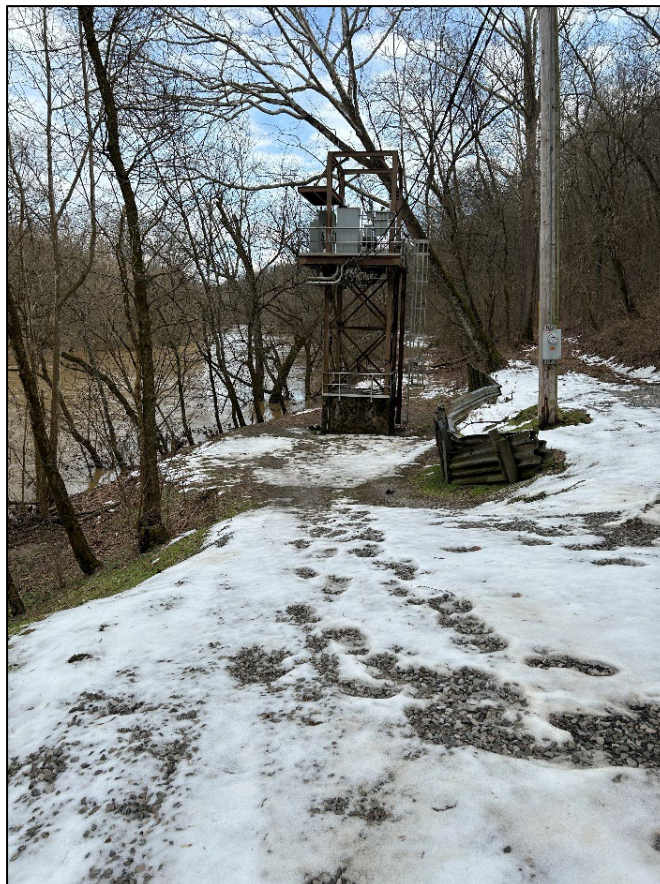
Photo: Cynthiana Water Works Licking River backup raw water intake
