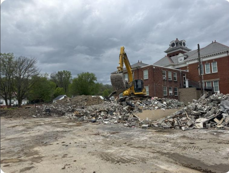
April 2026 – Site demolition and excavation work
