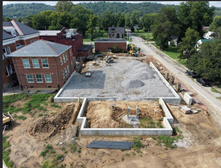
Foundation walls and preparing for block.
