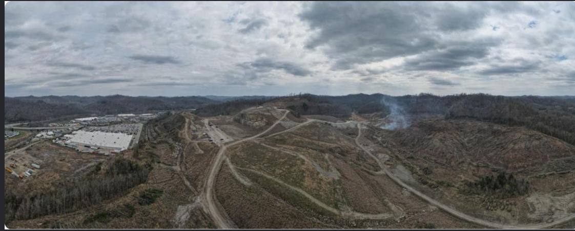
Site Development March 2023
