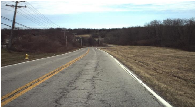
PATTERN CRACKING = Poor
