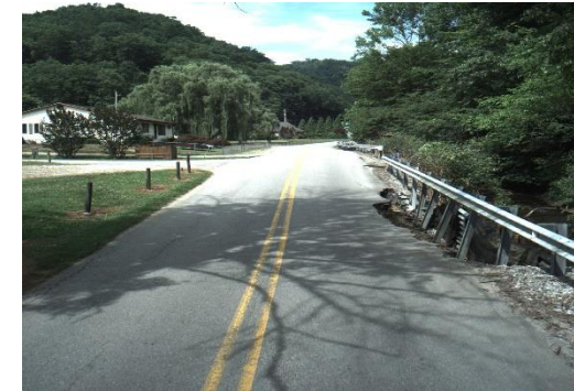
BASE FAILURE - Number
