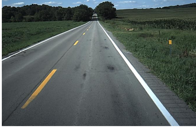
RUTTING = Poor
