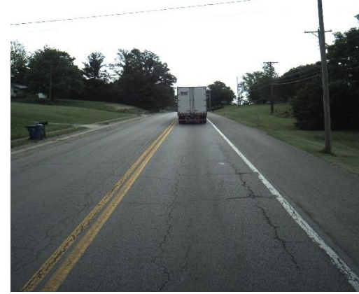
LONGITUDINAL CRACKING = Poor
