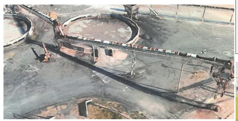
This project will remove the existing deteriorated conveyor system and reconfigure three 100' newly purchased 30" conveyors, install new bents, associated chutes and electrical power supply and controls. This project will ensure PMCRA can meet the barge unloading and delivery of more than 50,000 tons of fertilizer annually over the next 20-year period.
