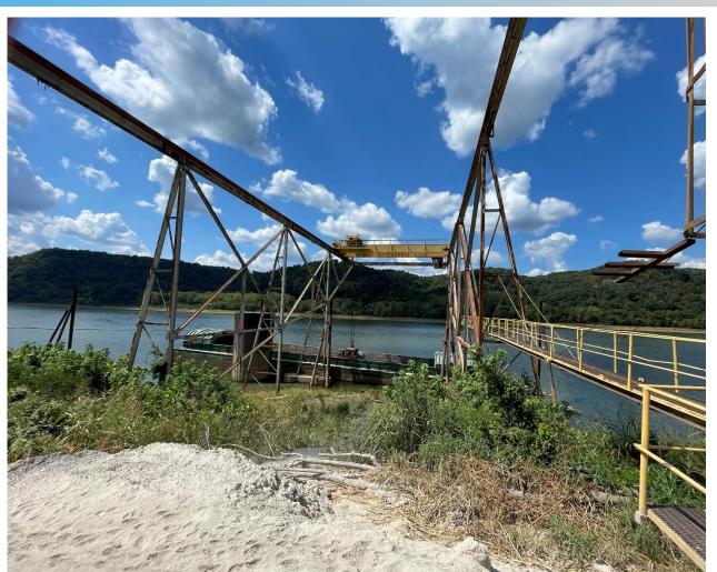
Project will replace 35-year-old gantry cranes electronic power, command control, cab, and braking systems. Will also retrofit the crane gantry structure to accept additional load capacity and replace the 30-year-old bucket and hopper system.
