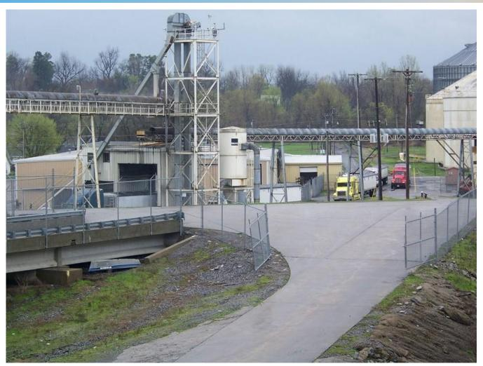
This proposed project would upgrade the Grain Truck Conveyor to allow for the eventual addition of a Hopper Surge Tank. The addition of the Hopper Surge Tank would hold grain until a barge is in position to accept grain. This will help eliminate long wait lines while the barges are moved. This part of the project will upgrade the pit conveyor and bucket lift to move grain to a future Hopper Surge Tank.
