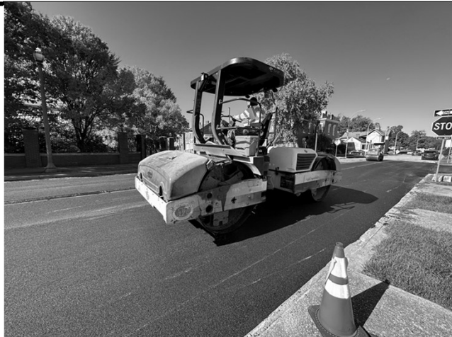
Source: Staff tour of H.G. Mays worksite.
