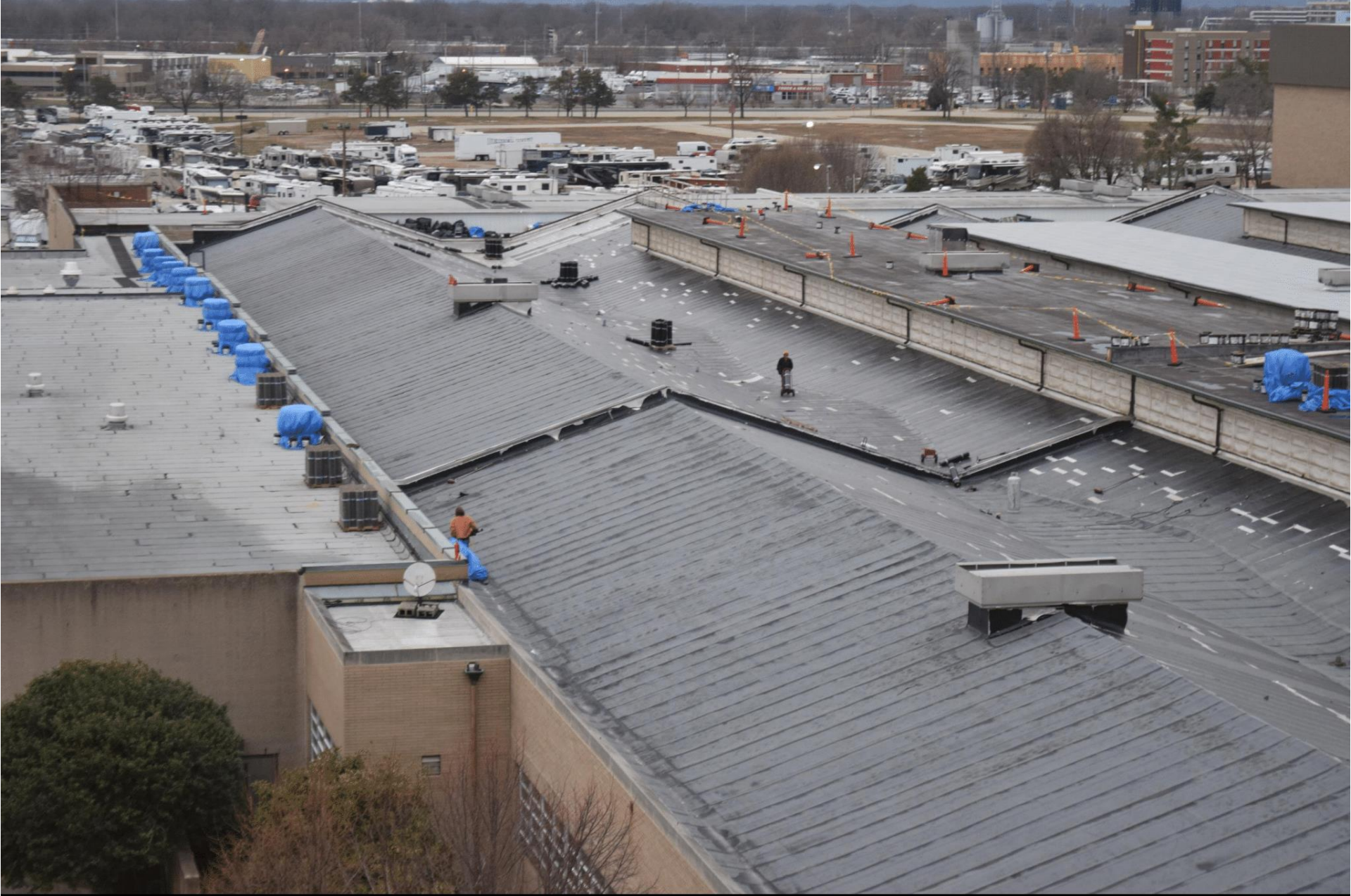
IN-PROGRESS West Wing Roof Repair
