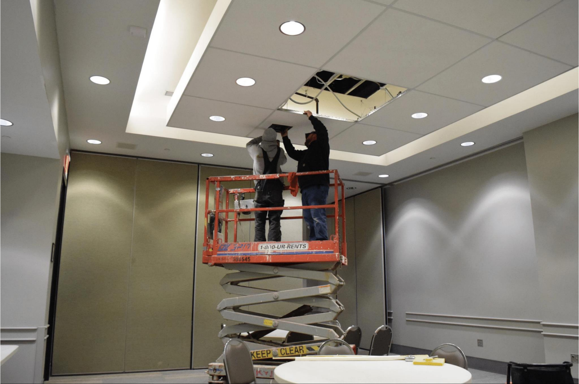
IN-PROGRESS: South Wing C LED Lighting Installation
