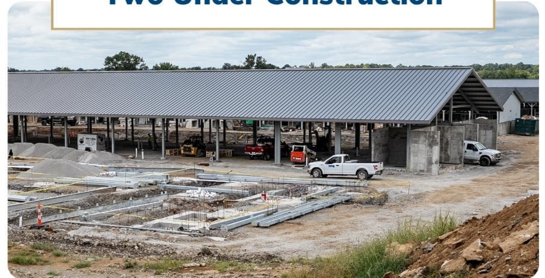
Two Under Construction
