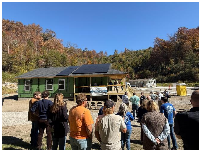
New home construction on Thompson Branch in Letcher County for flood survivors.
